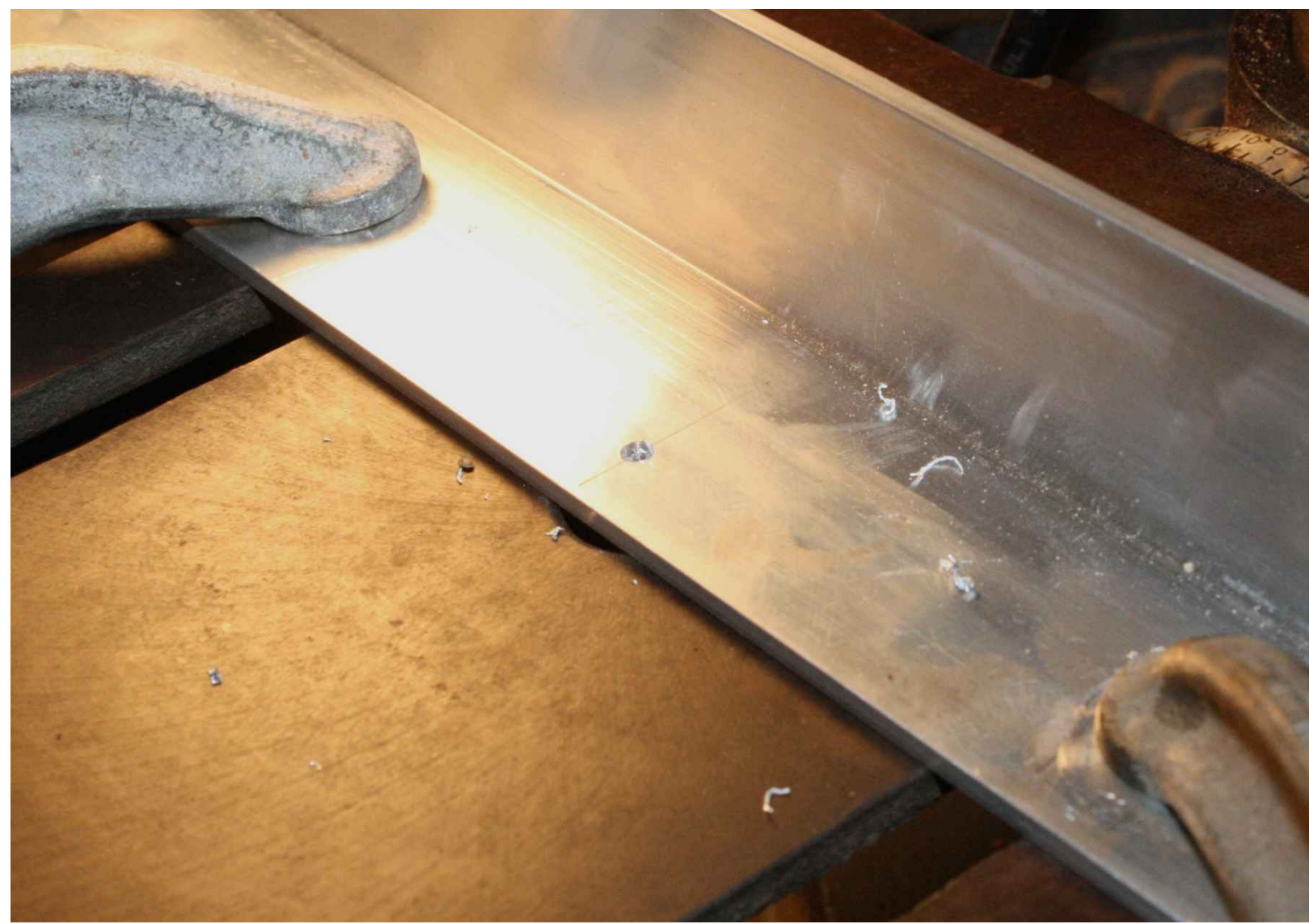
Figure 4-60. Drilled hole ready to tap
