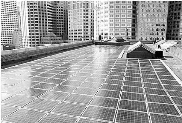
Figure 22.8 Powerguard flat-roof PV system including thermal insulation at the Coastguard building in Boston, MA (USA). The 3 kWp system has a special wind-tunnel-tested profile at the edge to keep the system on the roof in heavy winds. Adapted from Eiffert P, Kiss G, Building-Integrated Photovoltaic Designs for Commercial and Institutional Structures – A Sourcebook for Architects , 42–44, NREL, Golden, CO (2000). Reproduced with permission by NREL USA [18]
