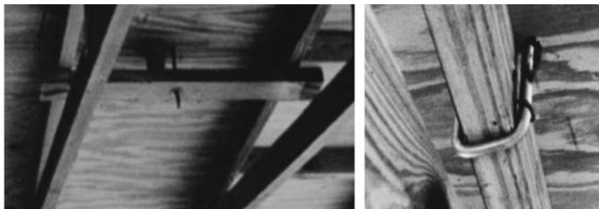
Figure 6.15 Spanner and J-bolt attachments provide secure anchors for roof-mounted arrays.
