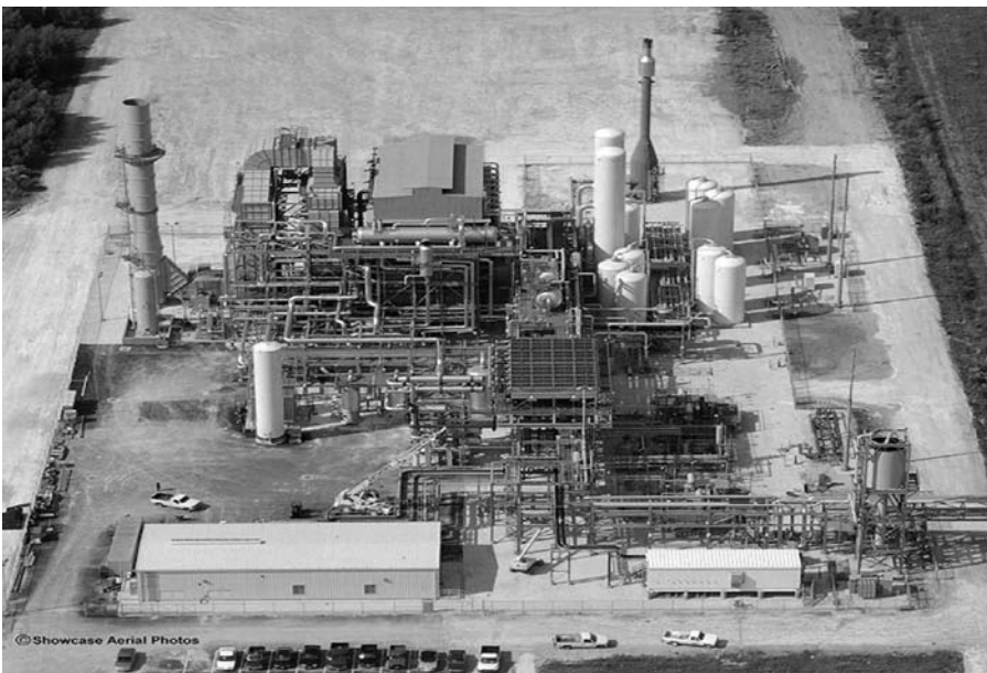
Figure 10.2. Aerial photo of Air Products and Chemicals, Inc.; an 80MMSCFD H 2 plant in Pasadena, TX (SMR H 2 facility and 10-bed H 2 PSA). See color insert.
