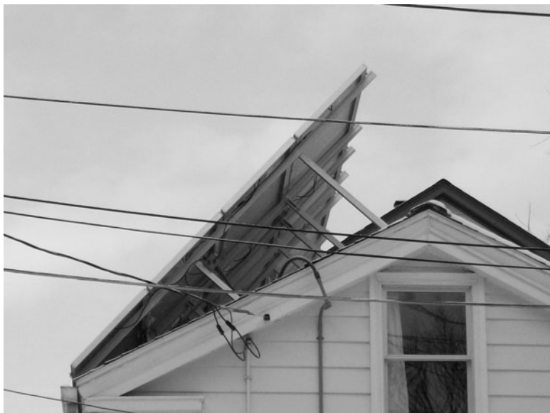
FIGURE 10-11 Roof-mounted PV array, Ithaca, New York, January 2007. Compare to mounting the PV rack flush to a gently sloped roof (see Fig. 10-8); the owner has incurred an extra cost to raise the angle of the panels, in order to improve productivity.
