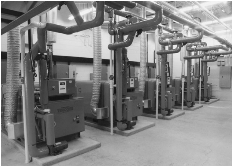
FIGURE 6-13 375-kW cogen installation using five Tecogen reciprocating generator units in Waverley, New York. Piping loops (red) connect hot water by-product to DHW, hydronic heaters, or absorption chillers. (Photo: Tecogen, Inc. Reprinted with permission.)
