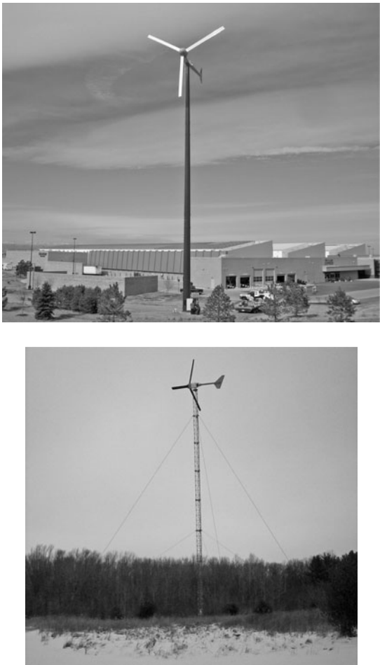
FIGURE 12-4 (a) Bergey 50-kW turbine on free-standing tower outside a retail center in Aurora, CO. (b) 10-kW Excel turbine erected on tower with guy-wires. (Upper Photo: Bergey Windpower Co. Reprinted with permission.)
