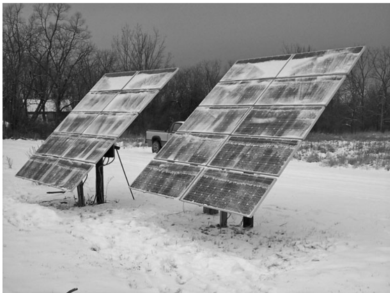
FIGURE 10-10 Ground-mounted 2.8-kW PV array near Mecklenburg, New York, January 2007. Ground mounting allows snow removal, and snow has just been swept from the panels at the time the picture was taken. Note that due to the overcast conditions, snow removal had only marginal effect at the time: with a thin cover of snow, the system produced 60 W, while in the condition shown it produced 120 W.
