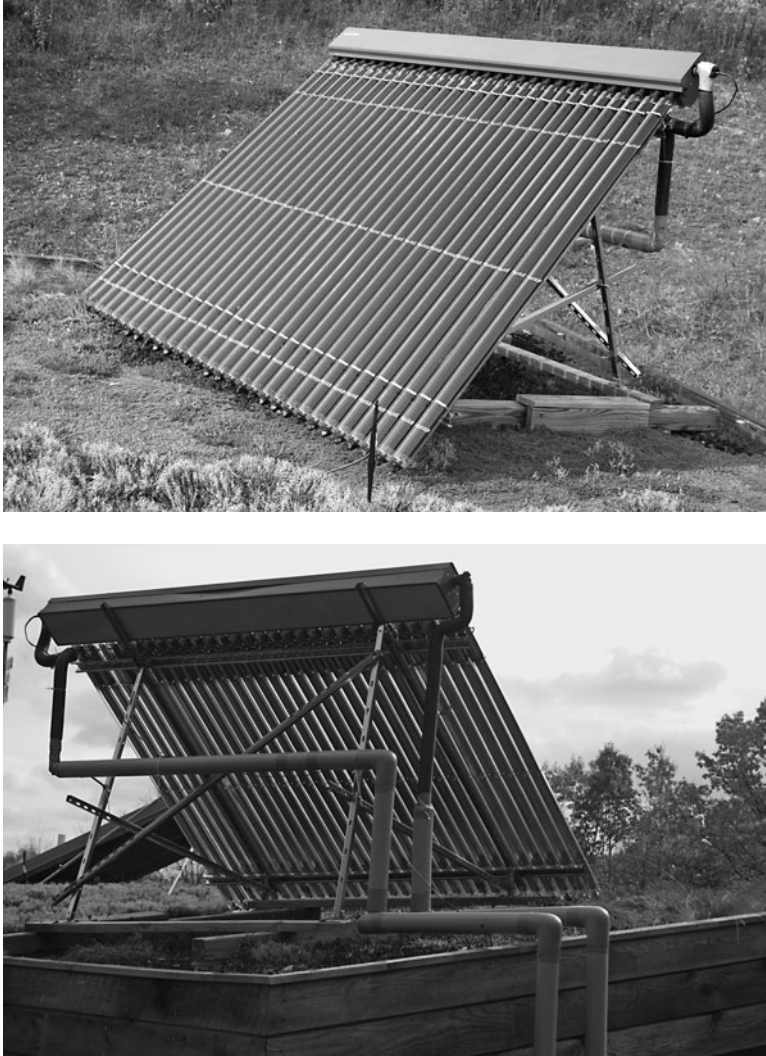
FIGURE 11-5 Evacuated-tube collector system
