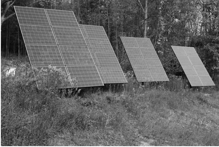
FIGURE 10-7 Ground-mounted PV array. Ground mounting permits seasonal adjustment of array angle (higher angle in winter, lower angle in summer). (Source: Philip Glaser, 2007, philglaserphotography.com. Reprinted with permission.)
