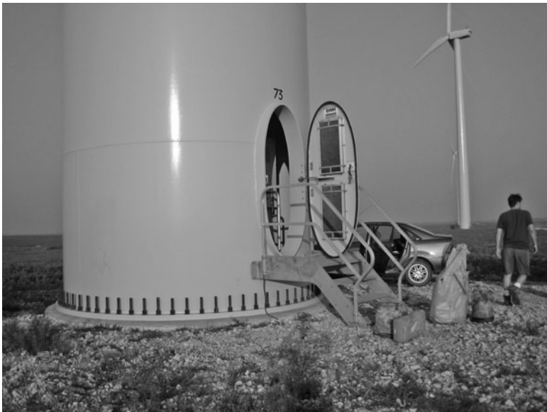
FIGURE 12-7 Access to the turbine nacelle via doorway and stairwell inside the turbine tower. (Photo: Ellie Weyer, 2007. Reprinted with permission.)
