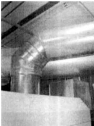
FIGURE 7-10 Indoor exhaust outlet. (Source: Elliott Energy Systems, Inc. 2004. Installation and commissioning manual EESI # 30. Elliott Energy Systems, Inc. Stuart, FL.)
