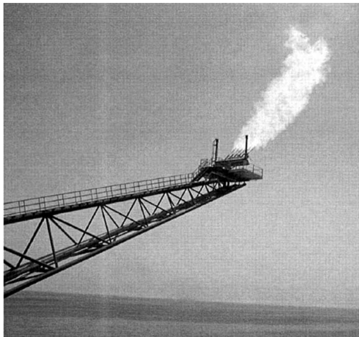
Figure 15.54 Water-assisted flare on an offshore platform. (From Ref. 63. Courtesy of John Zink Co. LLC.)
