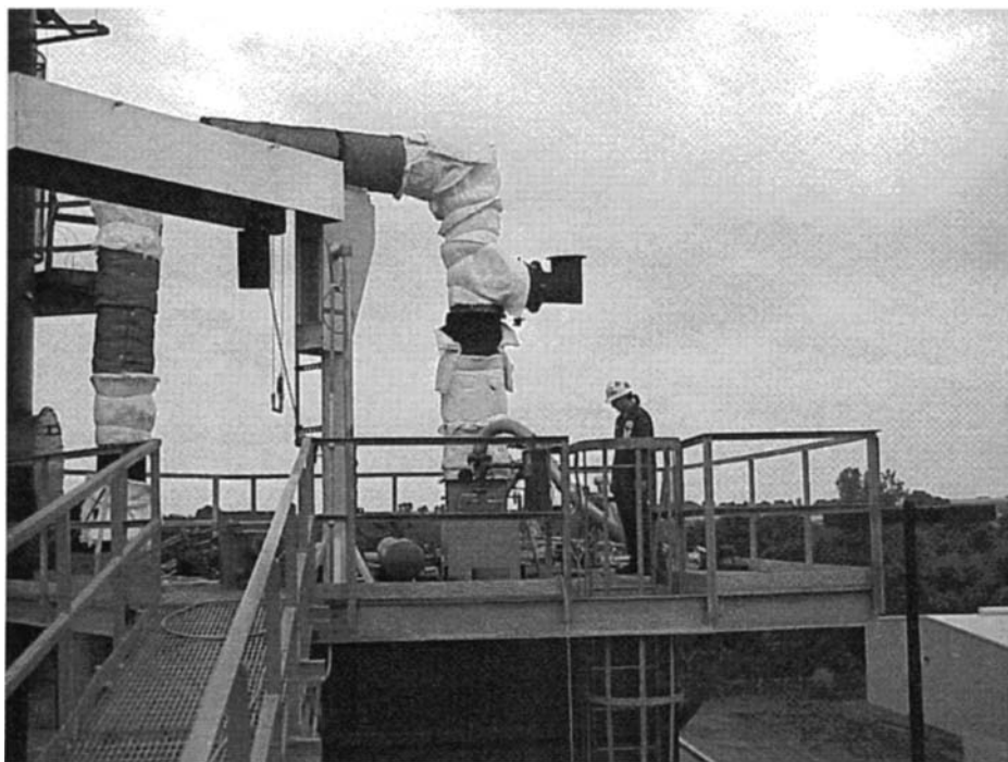
Figure 12.2 Example of a downfired, forced-draft, preheated air burner used in reformers. (From Ref. 2. Courtesy of John Zink Co. LLC, Tulsa, OK.)
