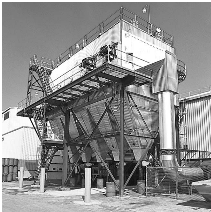
Figure 1.29 Photograph of a dry electrostatic precipitator. (Courtesy of United McGill, Columbus, OH.)
