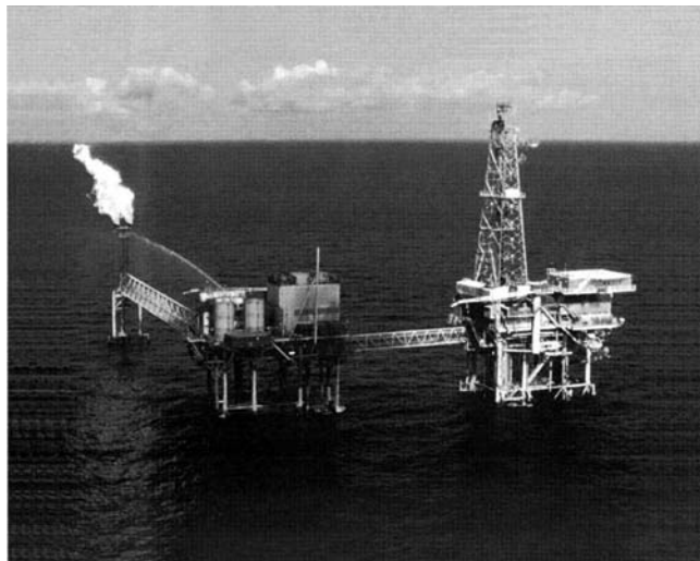
Figure 15.36 Radiation from an offshore flare. (From Ref. 63. Courtesy of John Zink Co. LLC.)
