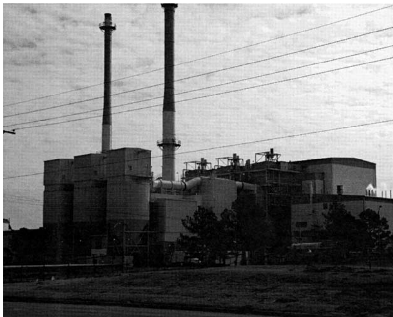
Figure 16.14 Municipal waste incineration plant.
