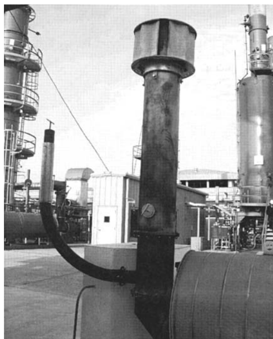
Figure 10.13 Quarter-wave tube installed on the exhaust stack of a propylene vaporizer: (top) front view; (bottom) back view. (Courtesy of John Zink Co., Tulsa, OK.)
